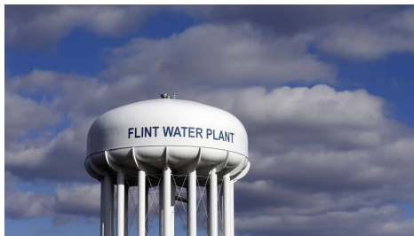
Figure 3: Flint Water Plant water tower (Osorio).
